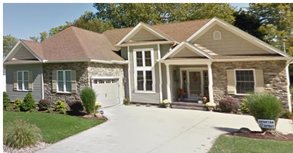
New Housing Construction
