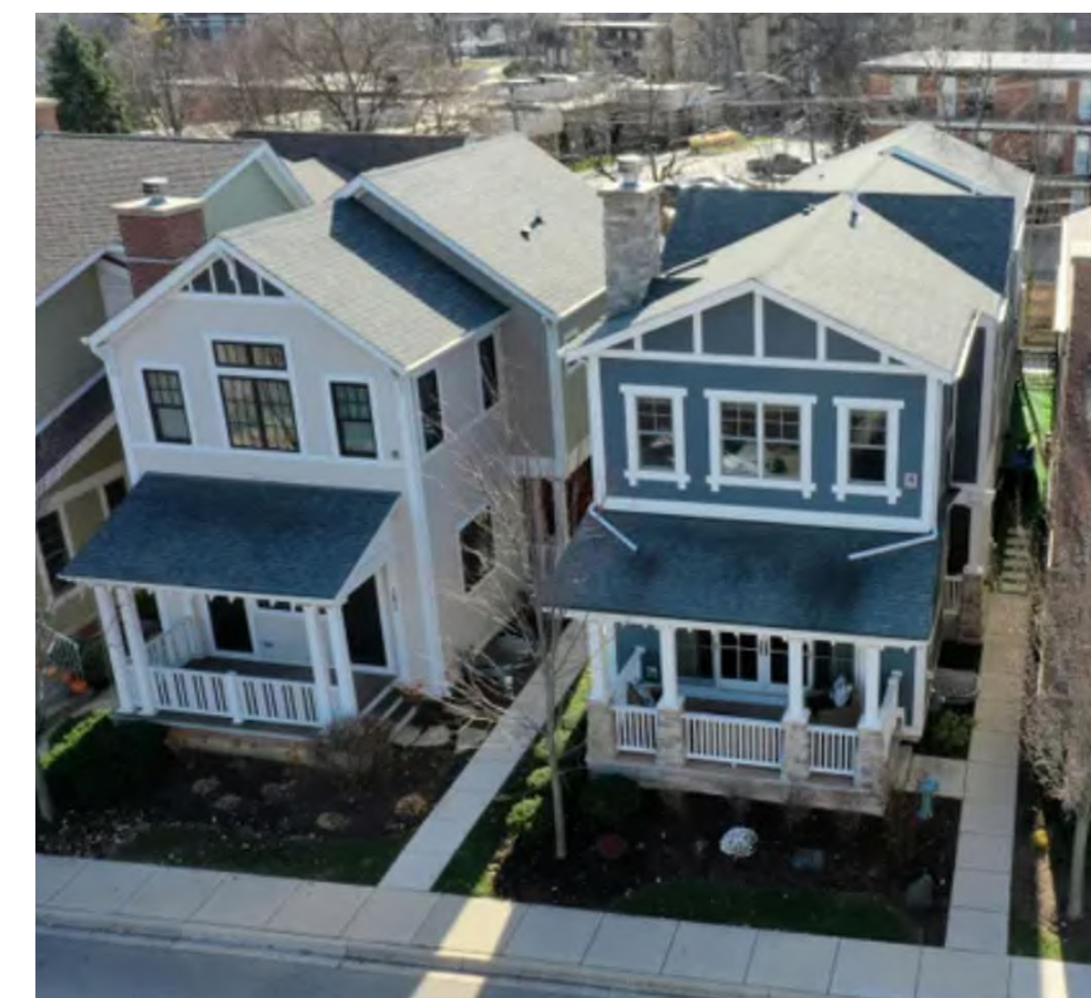
Dense development along Naylor Drive could consist of mixed-use two-story buildings on 50'x100' lots
