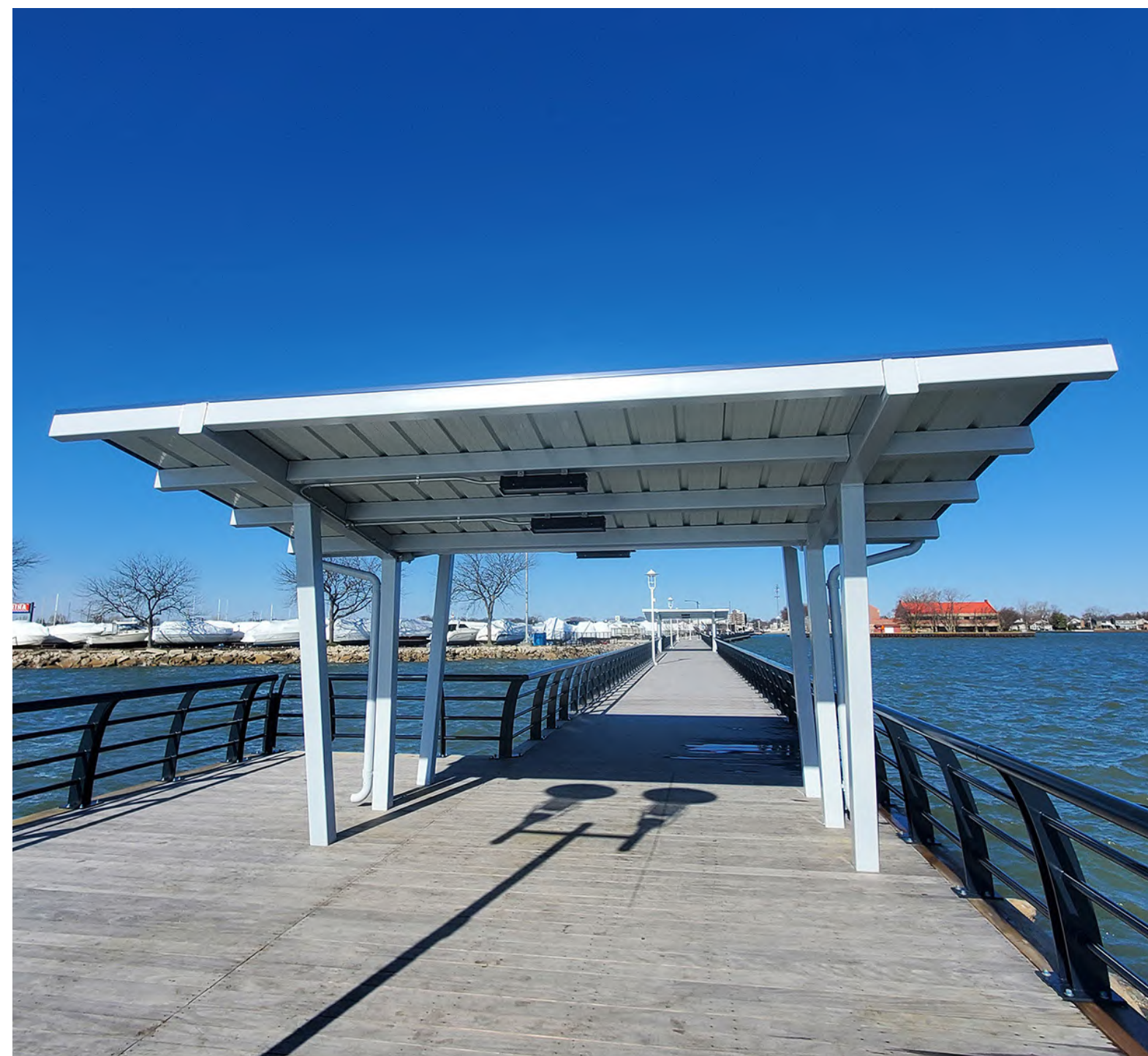
An iconic shelter will anchor the end of the promenade and frame views to the lake beyond
