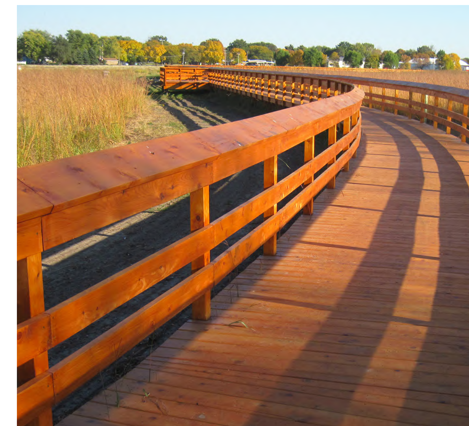
A cedar boardwalk through a wetland in Oregon, IL
