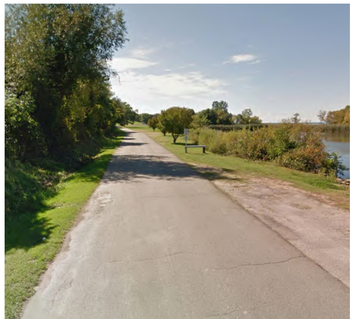
Naylor Drive is too narrow to safely accommodate pedestrians and cyclists
