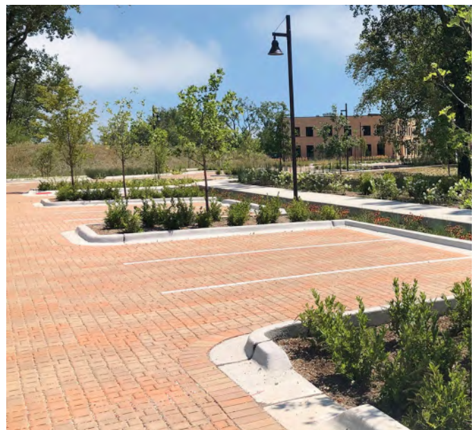
A mix of permeable paving and bioretention practices will detain and treat runoff from the expanded Naylor Drive
