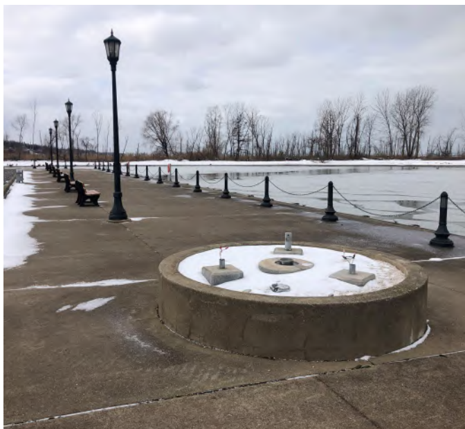
Visitors would benefit from better pedestrian access to the strolling pier
