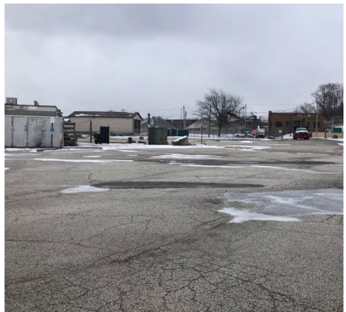
The lack of efficiently marked spaces limits parking availability and increases hazards for pedestrians
