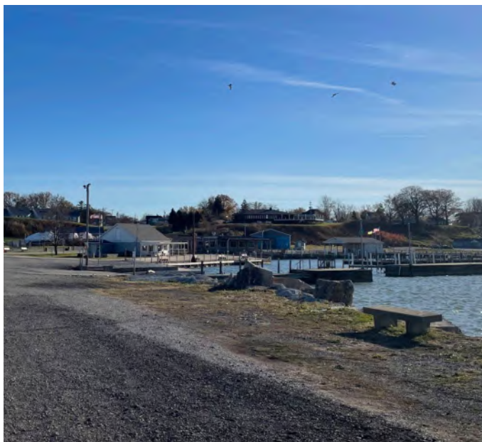
Stormwater runoff from the Marina Drive extension sheet flows directly into Lake Erie
