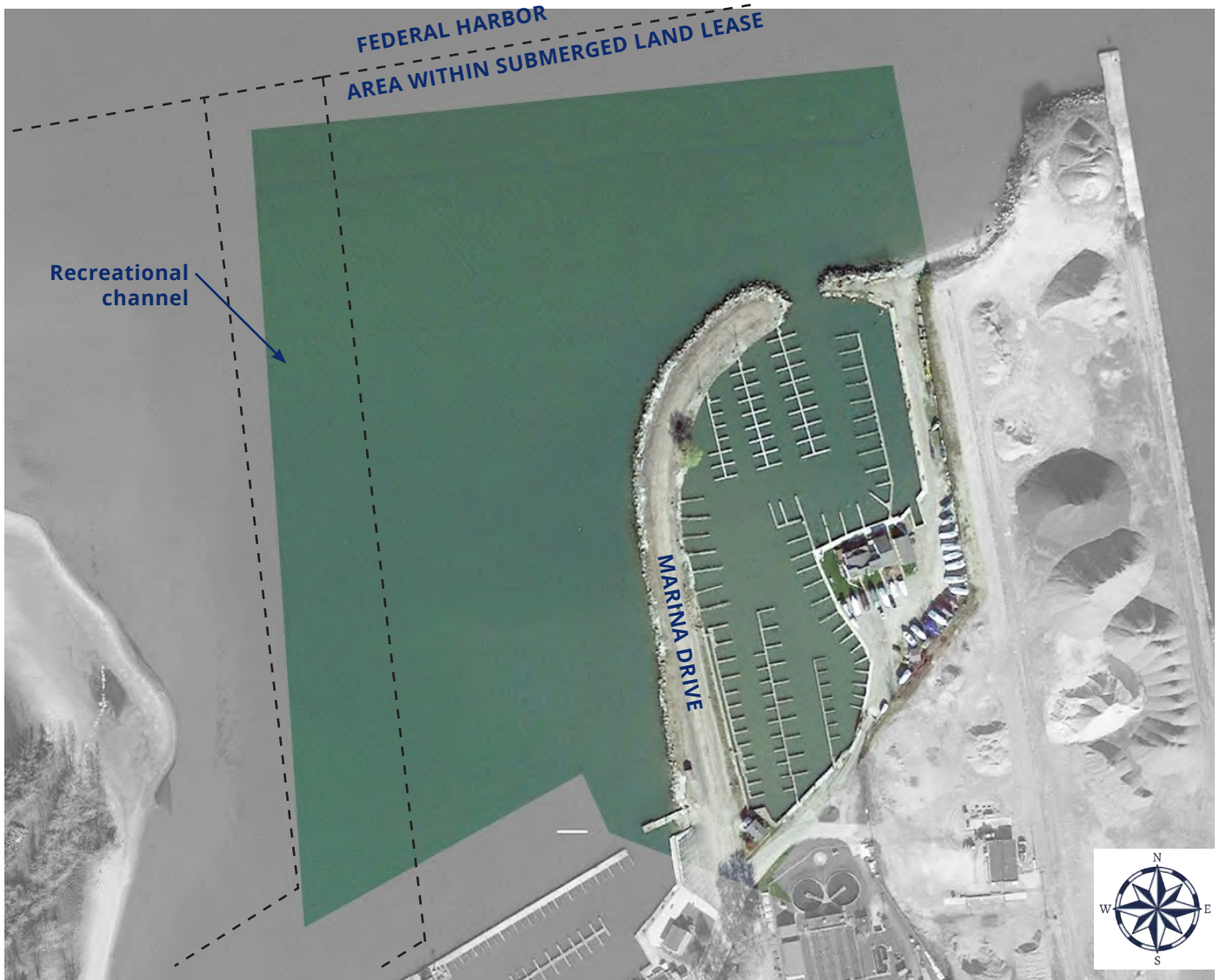
Aerial View of the Marina Drive Extension
