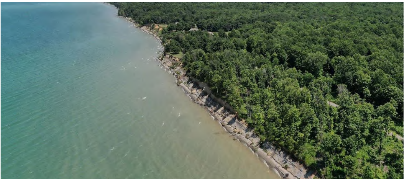
Beach nourishment projects would benefit the shoreline east of the port
