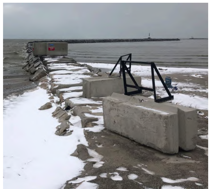
Unightly barriers have been installed at the breakwater to prevent access
